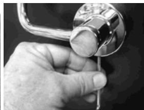
Tighten or remove using Allen Key
